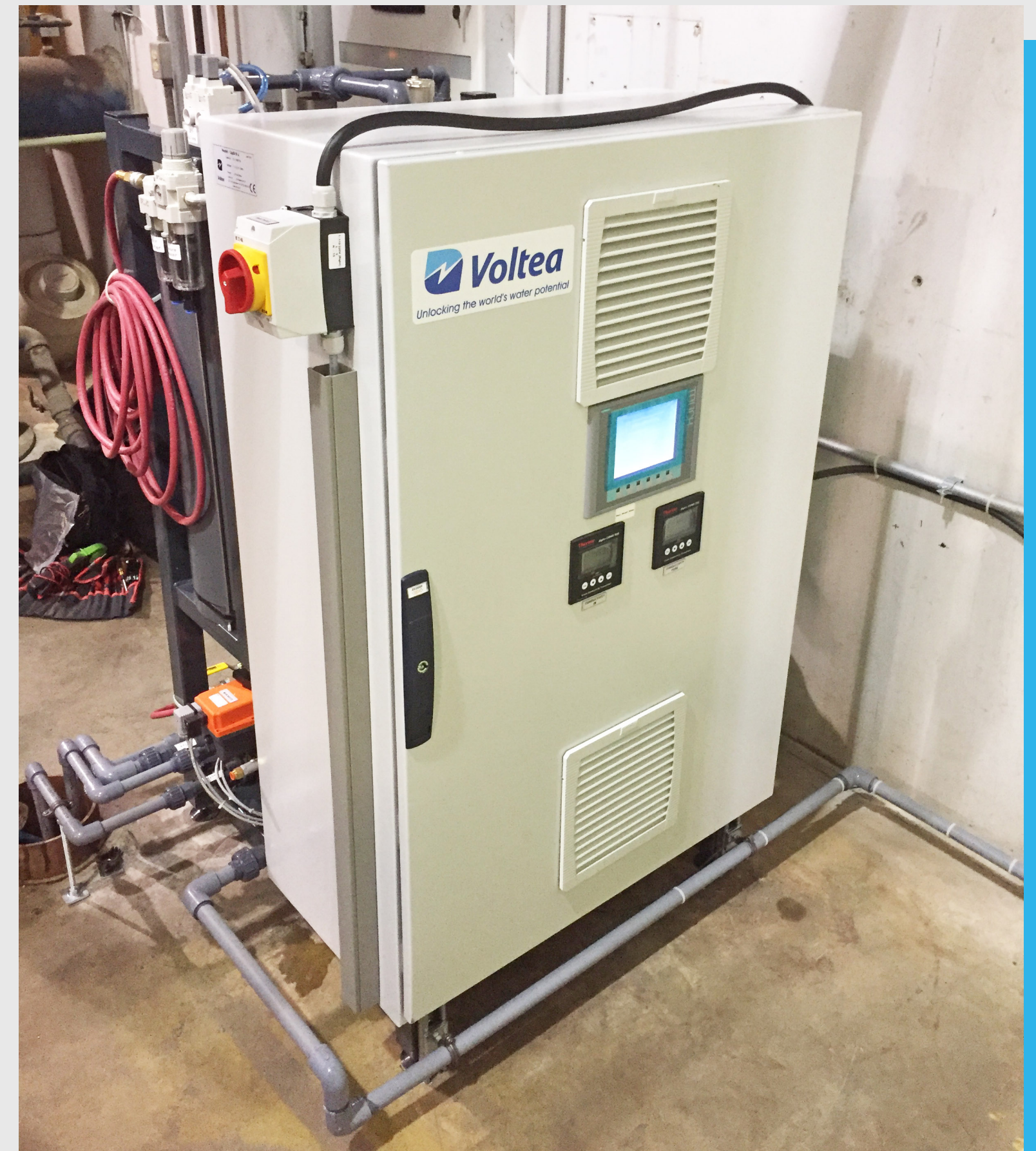
Voltea's Industrial Series 2 (IS-2) CapDI System on-site at Kalida Manufacturing
