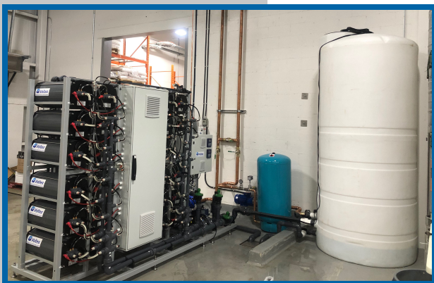
Voltea's IS-24 CapDI water purification complete with pressure and storage tanks at Wellington Brewery
