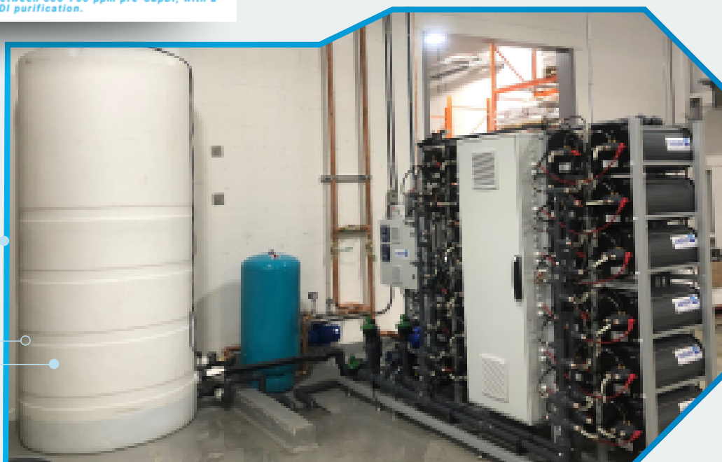
Figure 1 – Wellington Brewery feed water TDS hovers between 600–700 ppm pre-CapDI, with a target TDS of 125 ppm with CapDI purification.
